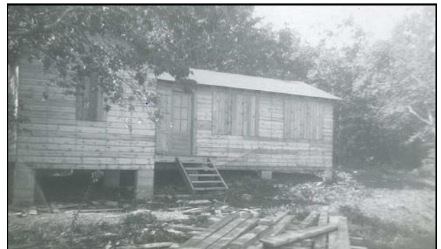
Eagle—Talon cabin being built
